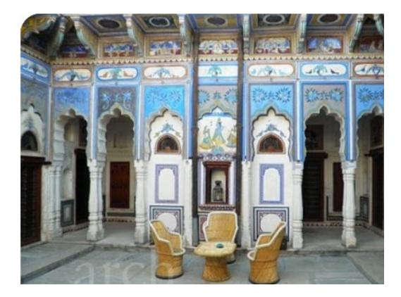
Courtyard was also an important design element in old residential buildings in hot dry climate including palaces. It was an element of passive cooling for regular fresh air supply and for day lighting. These interior courts - a common feature of Rajasthan architecture - optimize circulation of air during the 50°C summers. The rooms around courtyard are comfortable for use.
